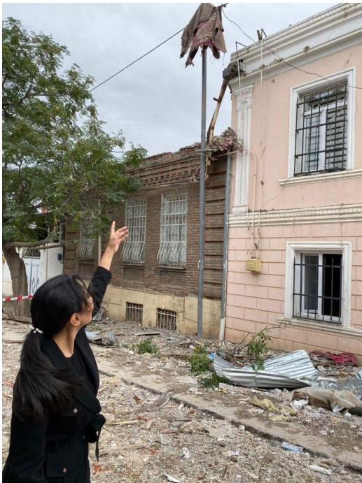
Destroyed private house – Photo 2.
